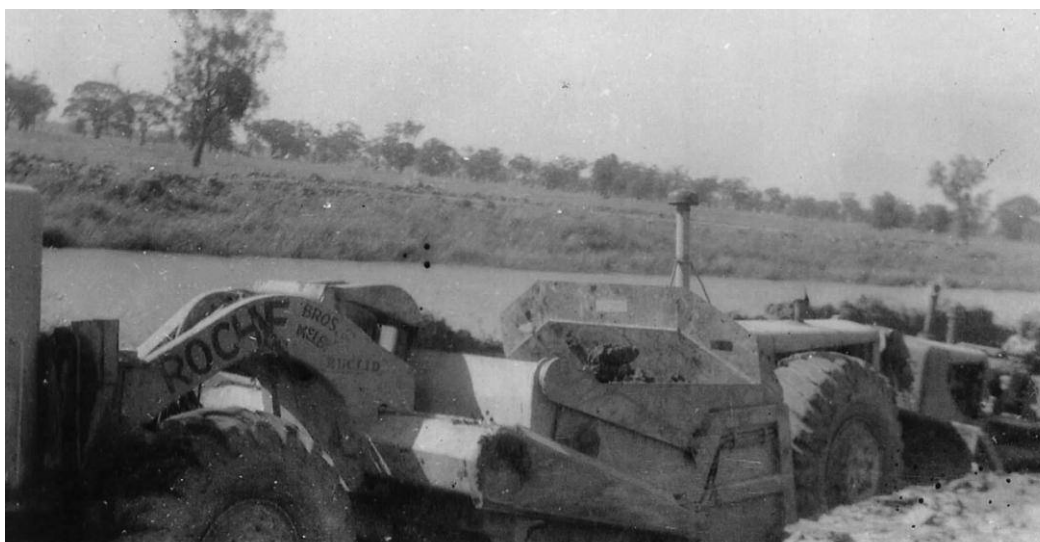
Euclid Twin Powered Scraper being pushed with an Allis Chalmers HD16.
