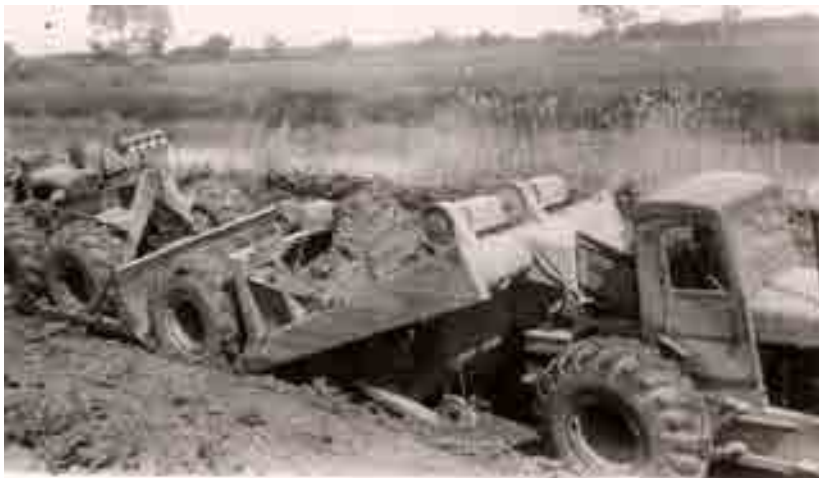
LeTourneau scraper powered by 6-71 GM. Scoop and steering were controlled with electric motors, and small toggle switches. They were pushed by a LeTourneau dozer also with 6-71 GM motor. Sub-contractors to Roche Bros 1956
