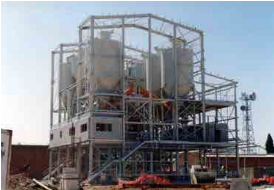
CSR Readymix Artarmon Plant , Twin Shaft Mixers and WAM Screw Conveyors and Cement Weigh Hoppers before it was fully clad as the plant below
