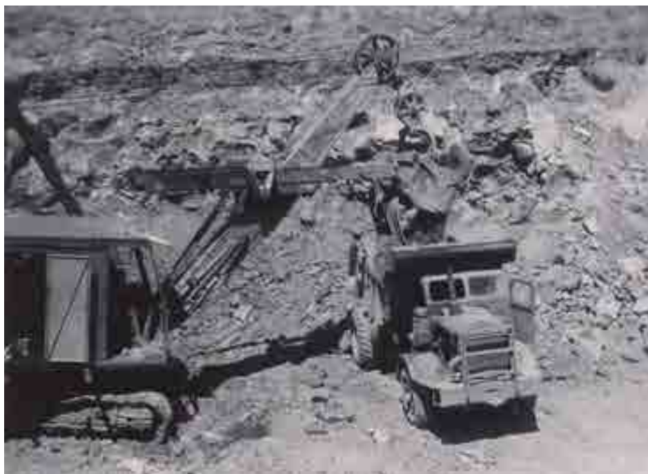
Face shovel loading beaching stone from spillway onto Euclid Trucking Co end dumper, Tallaroop Reservoir.
