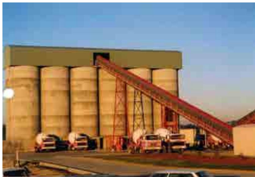
CSR Readymix Artarmon Plant , Twin Shaft Mixers and WAM Screw Conveyors and Cement Weigh Hoppers before it was fully clad as the plant below
