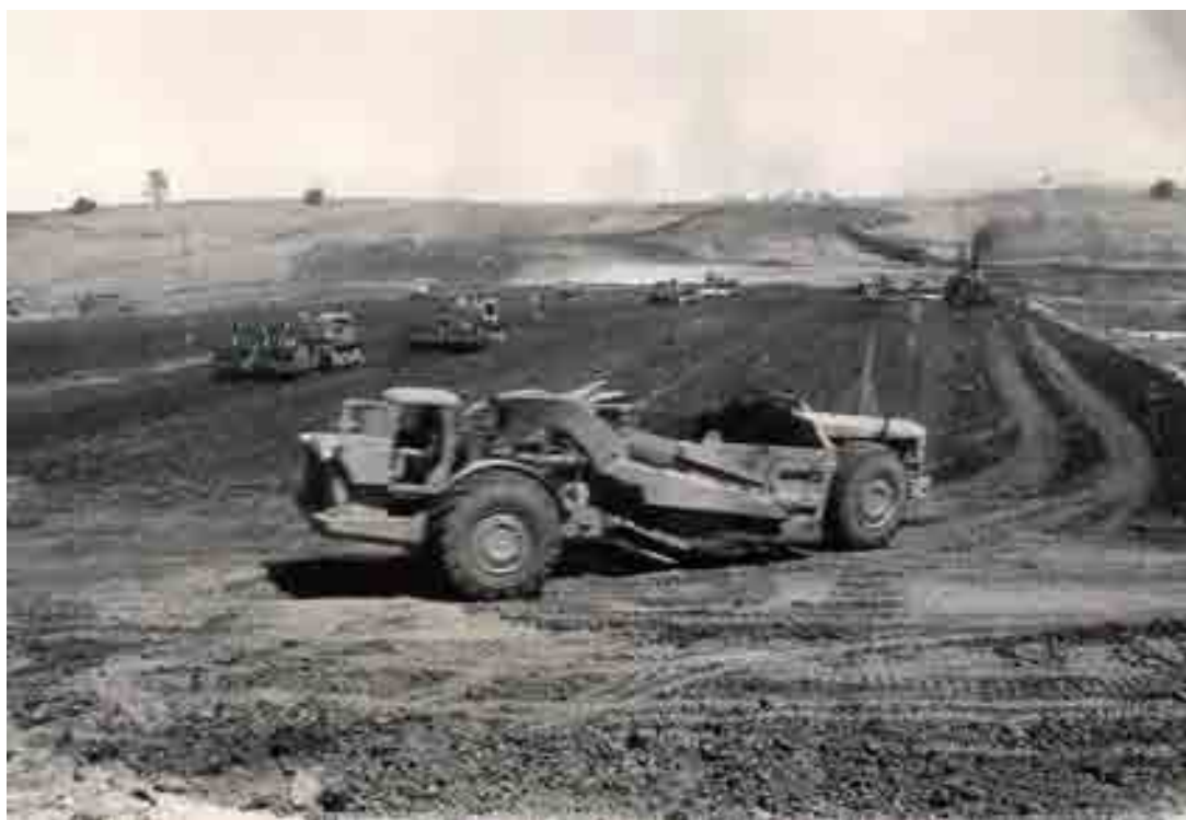
Max Currie's TS24 Euclid on main bank at Tallaroop Reservoir, also Euclid end dumper far left and belly dumper far right. 2 AC HD 20 pulling drawn sheep foot rollers centre. - Spillway excavation at rear.
