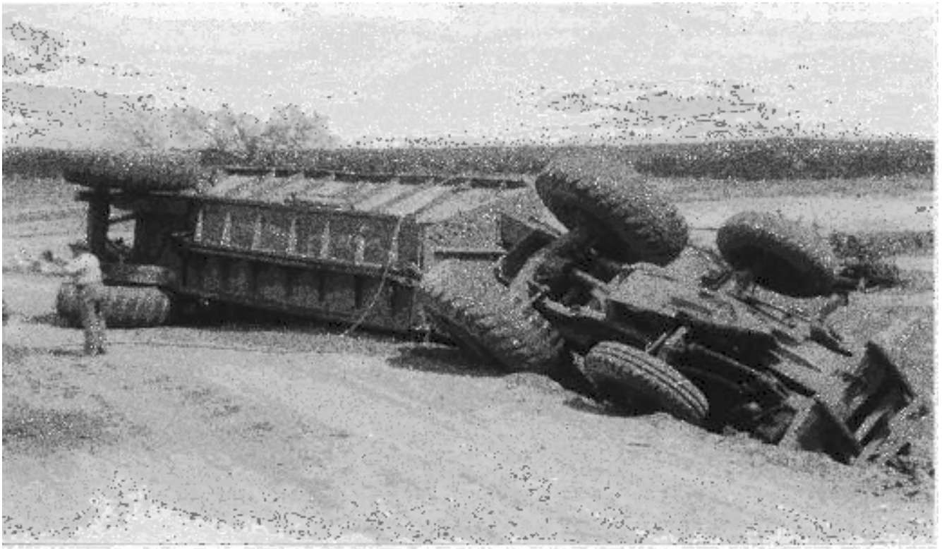
Euclid belly dumper in embarrassing position with Jack Scholes backing in tractor to stand it up. These machines were very prone to tipping because of a high centre of gravity. The driver always was thrown clear, and I never heard of a serious injury.
