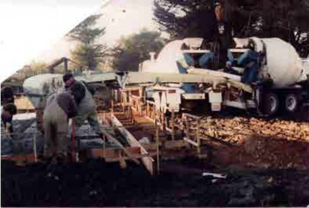
Terry Dwyer & Brian Simmons at Hislop and O'Meara building site at Latrobe Street, Kyneton placing concrete with a Theam concrete placement conveyor. We are Australian Agents for Theam.
