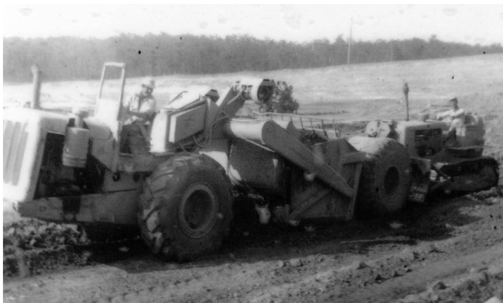
Thiess Bros Pup LeTourneau electric operated Tournapull scraper with 4 71 GM engine working at the Swanbank Powerhouse site being pushed with a Caterpillar D6
